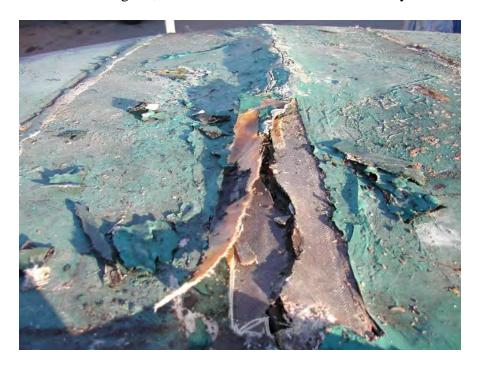
**Figure 10** Near top of door opening where upper and lower halves of shell are joined; vertical joint is connected with steel bolts, December 2002. Source: Milford Wayne Donaldson, FAIA.
