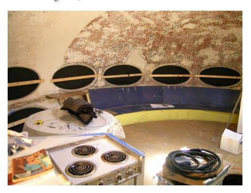
**Figure 16** Installing the mock-up acrylic window in a mock-up fiberglass frame made by Mr. Donaldson at Planet Plastics, Corona, CA, May 22, 2003. Source: Donaldson.
