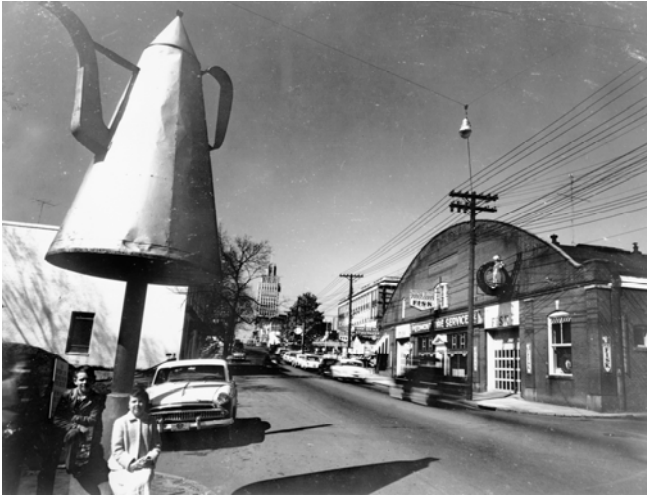
Highway construction at the Salem coffeepot, March 1956, in an image from the Forsyth County Public Library. Image courtesy of the State Archives, North Carolina Office of Archives and History.
